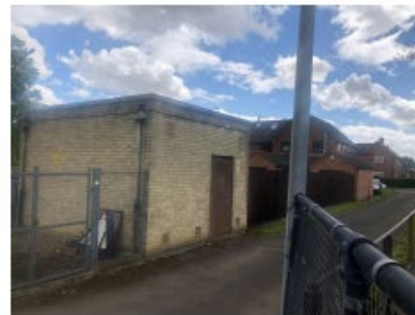
3. Existing Sub Station on perimeter of site
