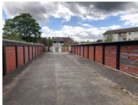
2. Existing garages on site
